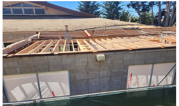
This picture shows the new framing above the offices.
