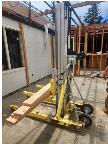
Genie Lift to move the lumber
