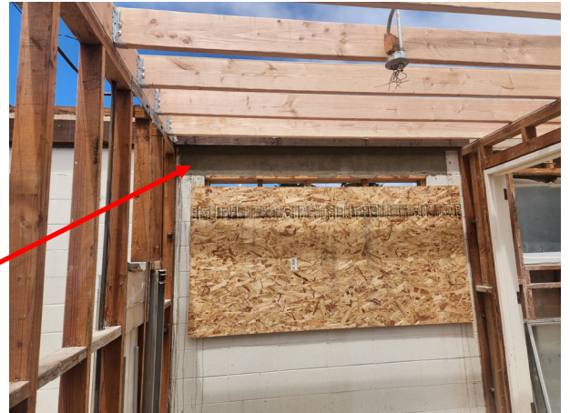
This picture shows the framing above the old women's restroom and the new header above the window that has been poured. See red arrow.
