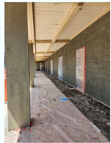
Classroom/Meeting Rooms Stucco—2nd (Scratch) Coat
