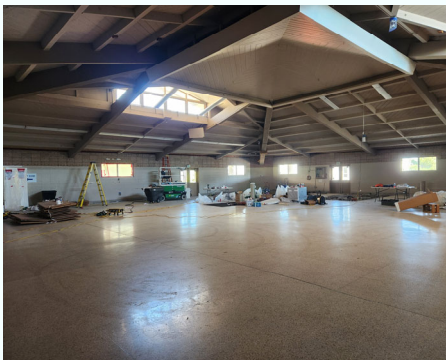
View of Hall from Kitchen Doorway Demo just beginning
