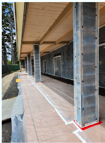
Classroom/Meeting Rooms Primer coat for stucco
