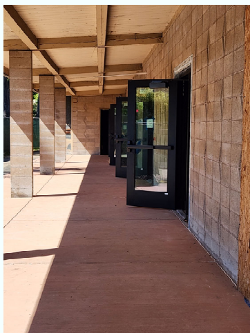
Classroom/Meeting Rooms New Doors, before Stucco
