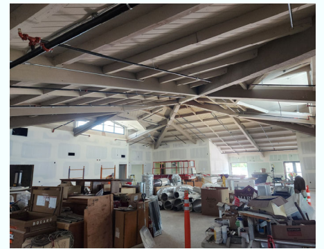
View of Hall from Kitchen Sheet rock is almost complete.
