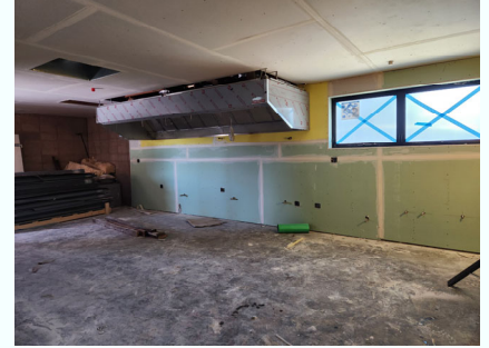
Currently—new hood installed & sheet rocked
