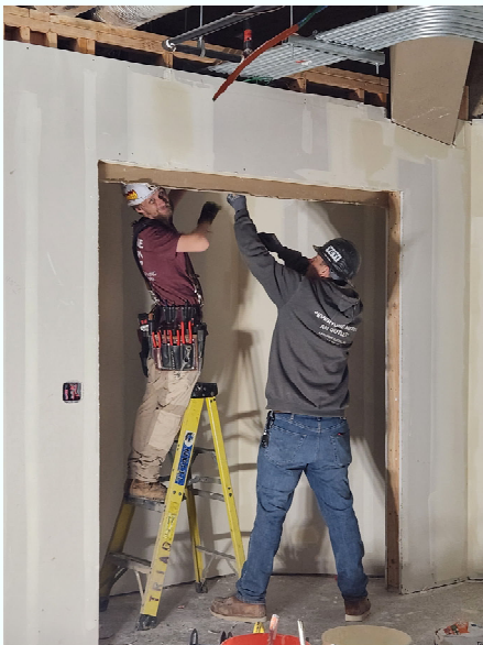
Pulling Electrical Wires
