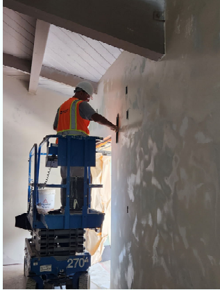
Texturing the Wall
