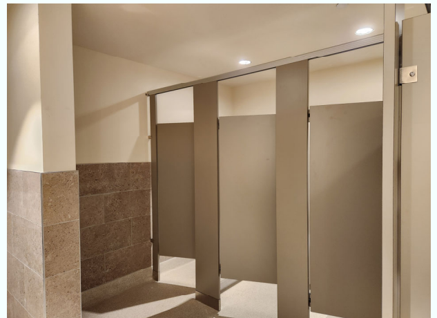
Sinks & Faucets are being installed in the restrooms Toilet partitions were installed.
