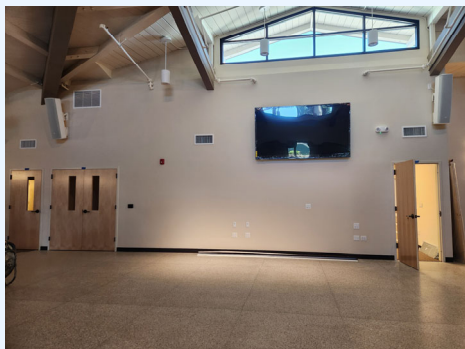
Speakers & Big Screen TV are installed.
