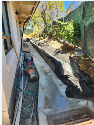
Drainage Work on the side of the hall
