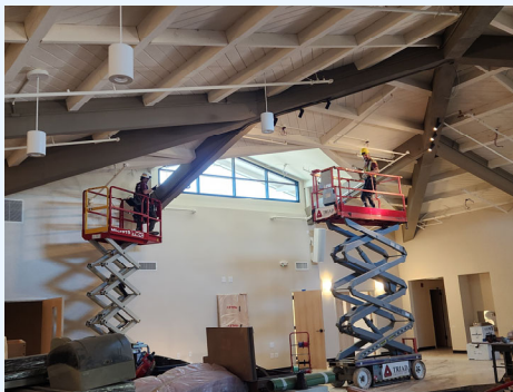
The pendant light installation continues
