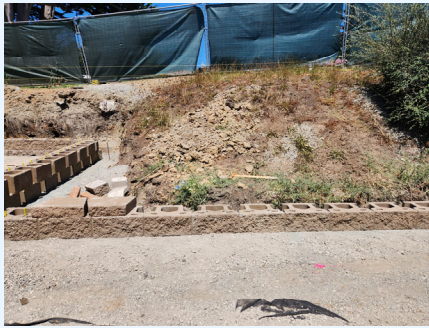
Retaining Wall is being installed behind the hall.
