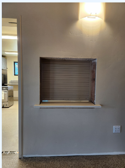
Coffee Station roll up door installed.
