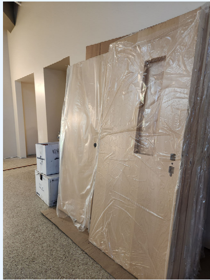
Interior Doors waiting for installation
