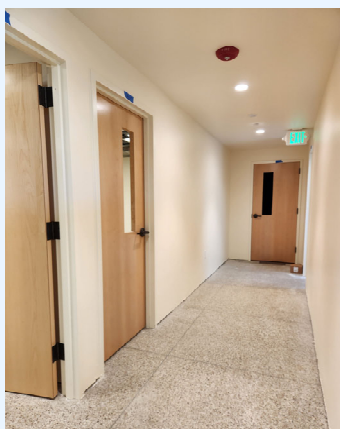
Interior Hallway with new doors & hardware
