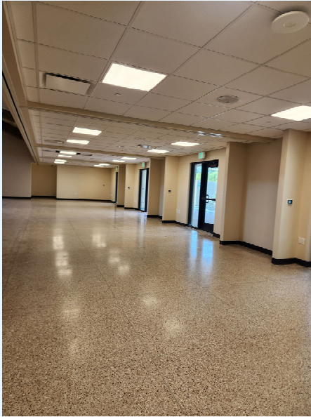
Drop Ceiling in Meeting Room/ Classroom Area
