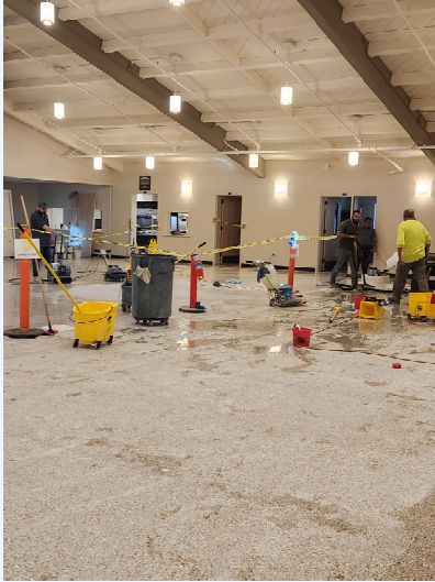
Working on the Terrazzo floors
